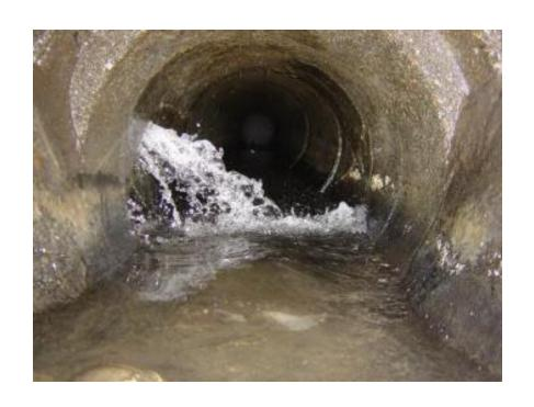
Sanitary and storm sewer piping is shown with a slope less than the minimum allowed by code
